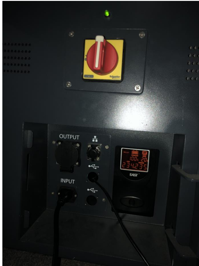
Figure3: Main Switch and User Service Panel
