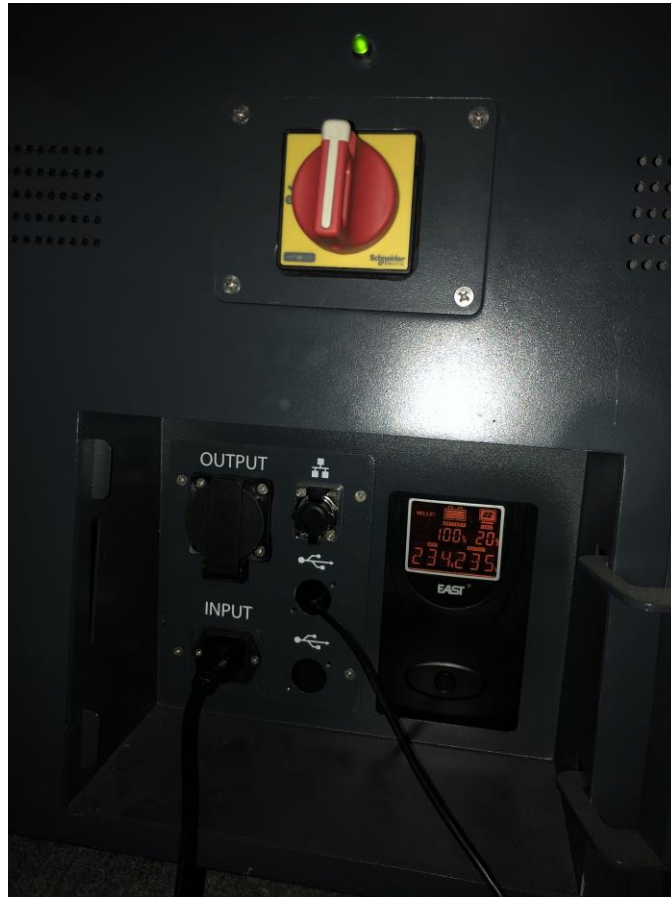
Figure3: Main Switch and User Service Panel
